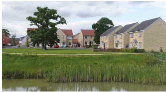
Sustainable Drainage Systems
